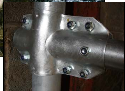
These are the new heavier clamps – all with a bolt though - cubicles and brackets are all hot dipped galvanized.
