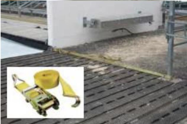
7. At the other end, stretch the top cover using a ratchet strap until the top cover is smooth and tight.
