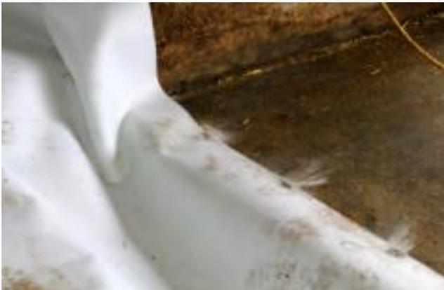
6. Fasten one end of the Top Cover using plastic strips and a few nailins.
