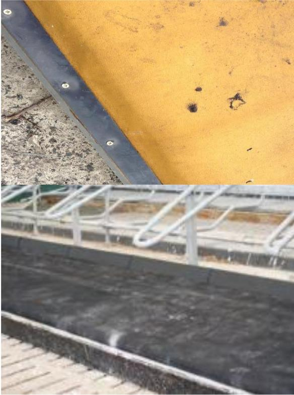
17. One top cover is tight, use plastic strip and nailins to hold it in place, using approximately 1 nailin for every 12" (30cm) of strip. Plastic strip is also used to fasten along each end of the mattress run
