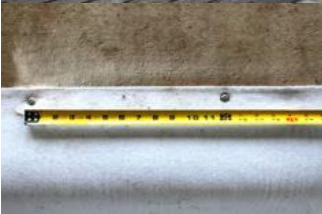
8. Go back to the first end and begin fastening down the top cover along the chalk line, using plastic strips and nailins (approximately 12" or 30cm apart).
