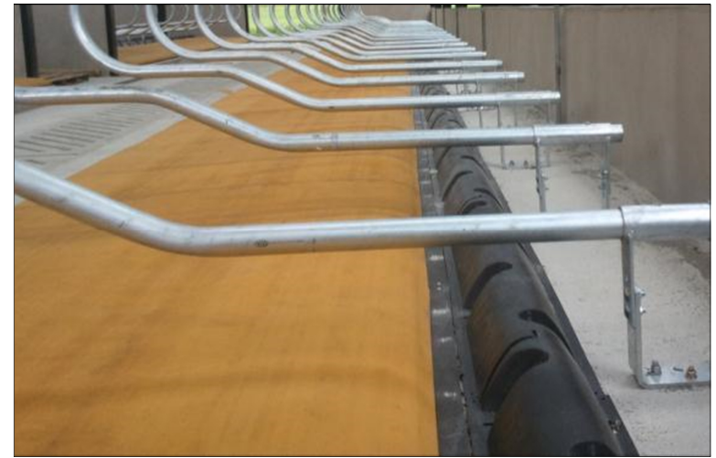
FIGURE 5. Pasture Mat mattresses installed with moovApillow (NOTE: sometimes the MoovApillow will overlap the plastic strips)
