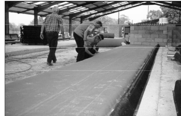
FIGURE 6. Tuck the top cover under the mattresses as tight as possible.
